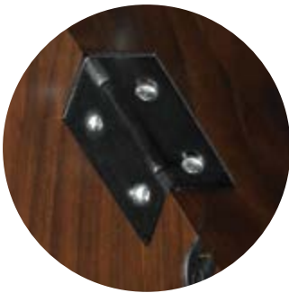
Tamper-proof brackets on all exposed connections
